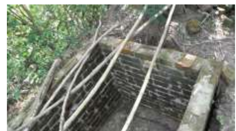
Baluram has already started to construct a latrine
