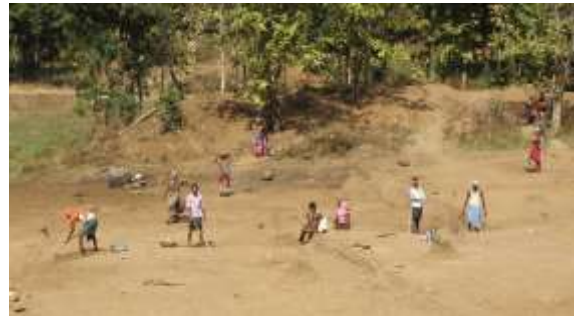
Villagers earning money while building for the future as they work on the check dam at Bikrampur
