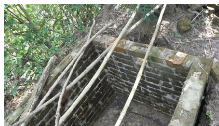
Baluram has already started to construct a latrine
